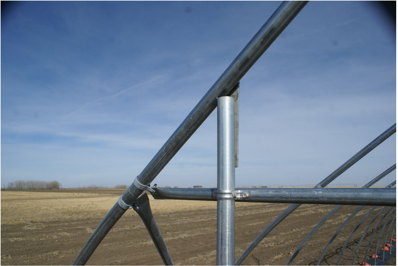
Picture 8: pipe straps are used to fasten the vertical end wall post to the horizontal cross brace of the end arch
